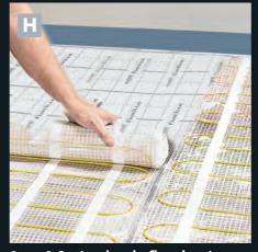
Stage 3 Optional underfloor heating Aqua-Mat® underfloor heating comes on a roll of webbed backing that can be laid over the entire floor. This can then be connected to a wall mounted thermostat.
