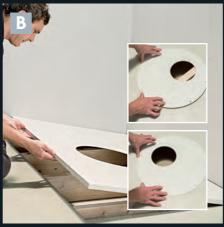
The Aqua-Dec EasyFit is then placed in the recess to determine where the waste needs to be fitted. The Aqua-Dec EasyFit, has unique drain features\* that allows it to be rotated to avoid any joists that could obstruct the waste.
