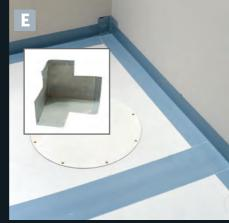
Corners are then sealed with the preformed Waterguard® corner pieces. Jointing Tape is then laid in 1m parallel strips.
