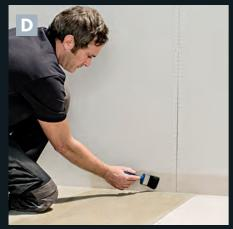
**Stage 2 Waterguard® Waterproofing**First, the entire floor (excluding Aqua-Dec EasyFit) and 75mm up the wall is painted with the primer. **DO NOT PRIME THE DEC**
