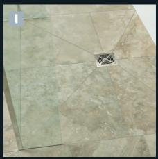
Stage 4 Tiling and wetroom glass panels For the shower area, larger tiles like these above will need to be cut diagonally to follow the gradient in the Aqua-Dec EasyFit. Alternatively, you can use mosaic or small tiles (max. size 50mm square), which will naturally follow the gradient.
