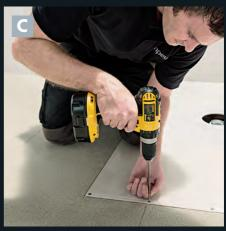
Once the waste is fitted the Aqua-Dec EasyFit can be screwed directly to the floor joists.
