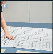
The Waterguard® membrane is then rolled out to cover the Aqua-Dec and THE ENTIRE FLOOR.
